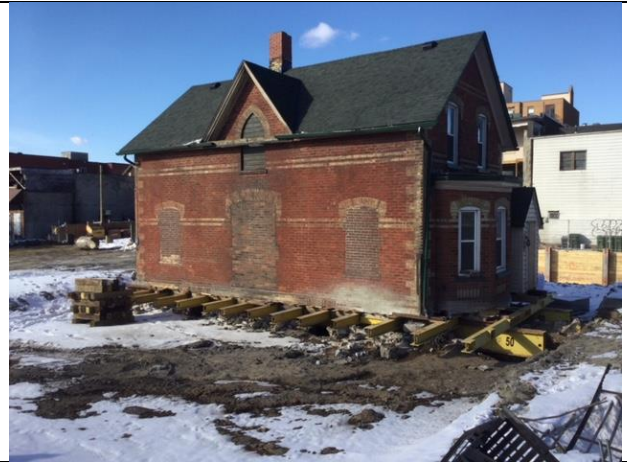
South and east elevations, January 30, 2021. Barbara Myrvold
