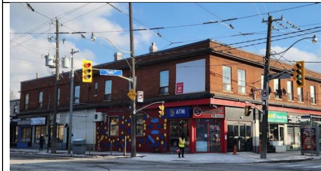
155, 161, and 167 Main Street and 2201-2207 Gerrard Street East. Built 1903. Representative of early-20 th century Main Street Commercial Block building. Valued for its association with the Snell family, significant in the early development of East Toronto.
