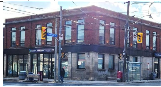
164 Main Street, southwest corner of Gerrard Street East. Built 1903. Representative of an early-20 th Main Street Commercial Block type building. Historically known as Snell's Hall, valued for its association with the Snell family, significant in the early development of East Toronto.
